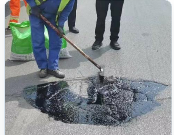
Fill and level
