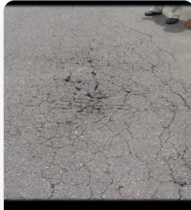
Cracked road surface repair
