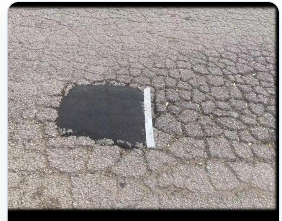
Completed patch area
