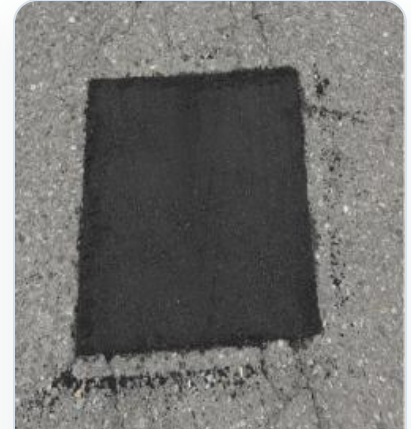
Finished repair surface
