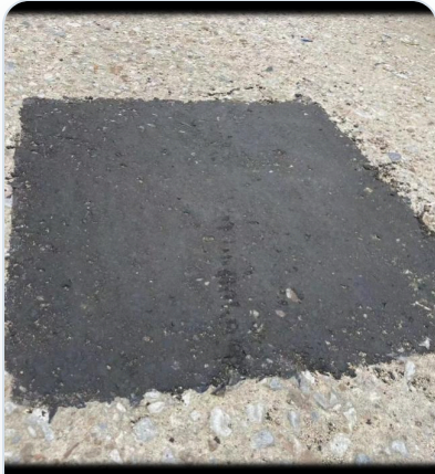
Local pavement repair
