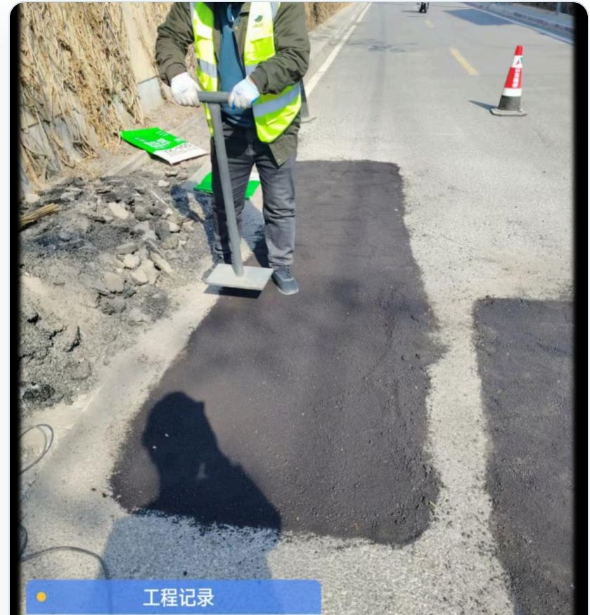
Final leveling before opening
