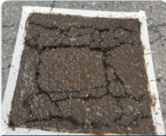
Fill the damaged section
