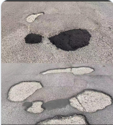
Pothole repair in asphalt pavement
