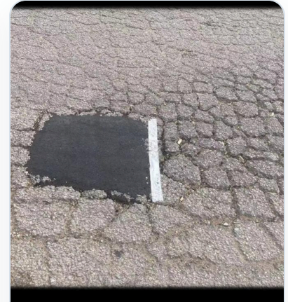
Completed patch in cracked area
