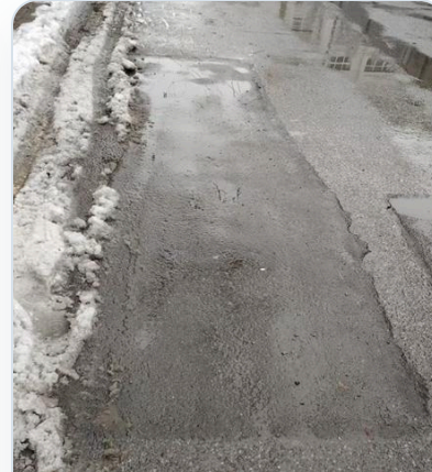
Wet road maintenance
