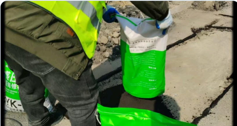
Material filling on site
