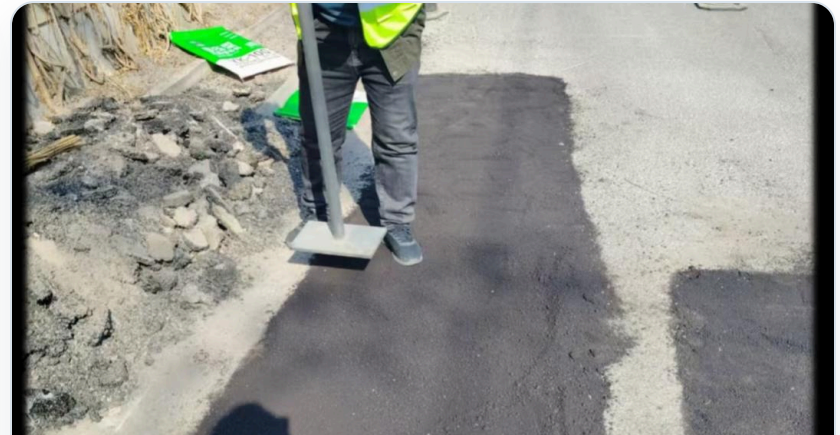
Manual leveling and compaction
