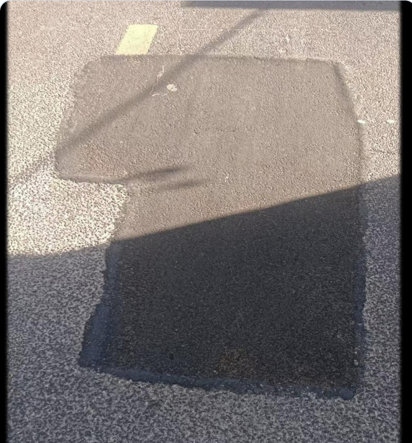
One-month repaired surface
