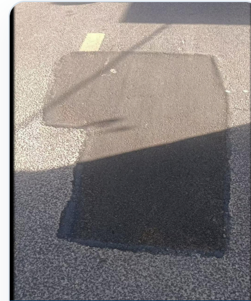
One-month repaired condition
