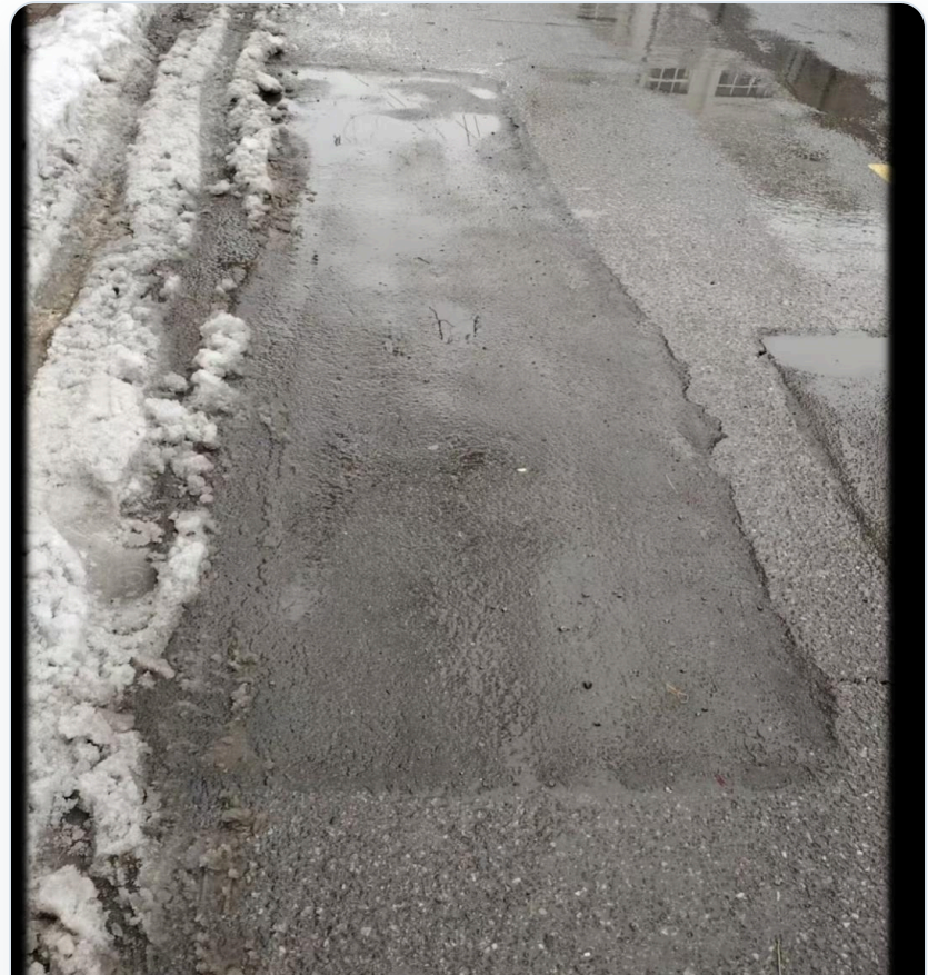
Repaired area remained stable
