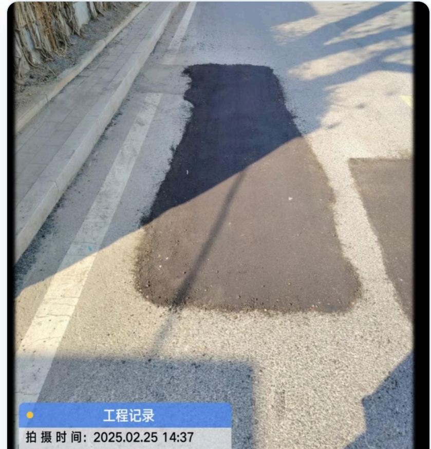
Surface under traffic use
