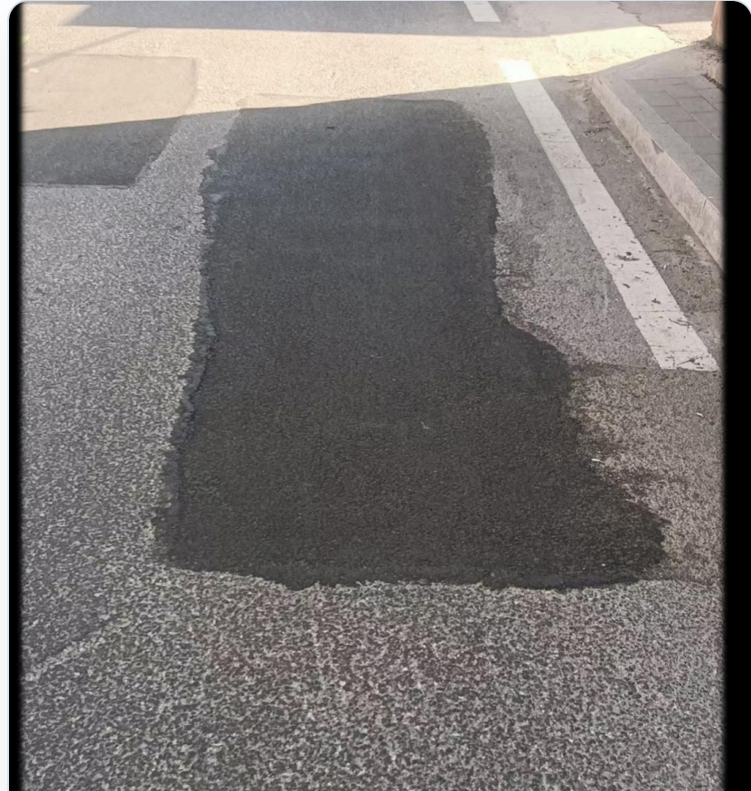
Stable road surface condition
